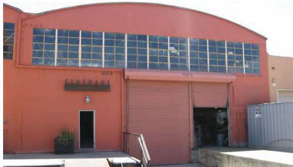
Adaptive reuse of historic buildings provides new opportunity for small business
