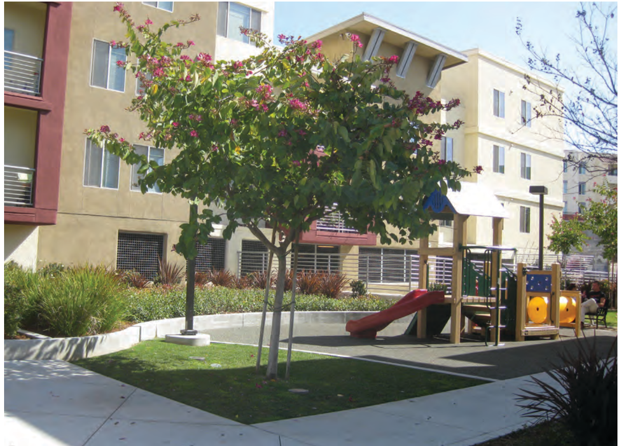
Orientation and configuration of development should allow for adequate access to light and air
