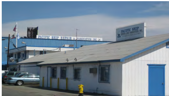
Pacific Ship Repair building
