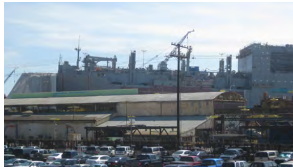
NASSCO Heavy Industrial
