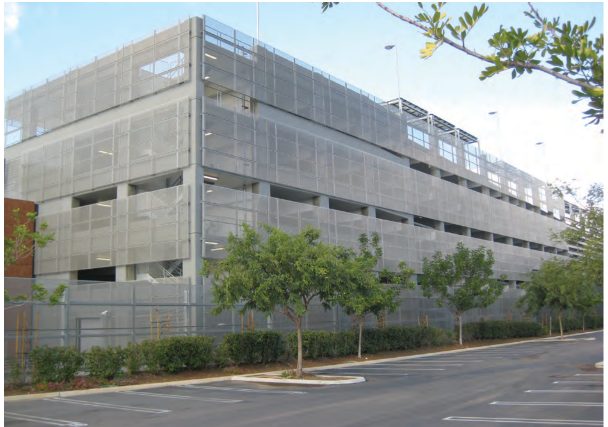
A typical parking garage
