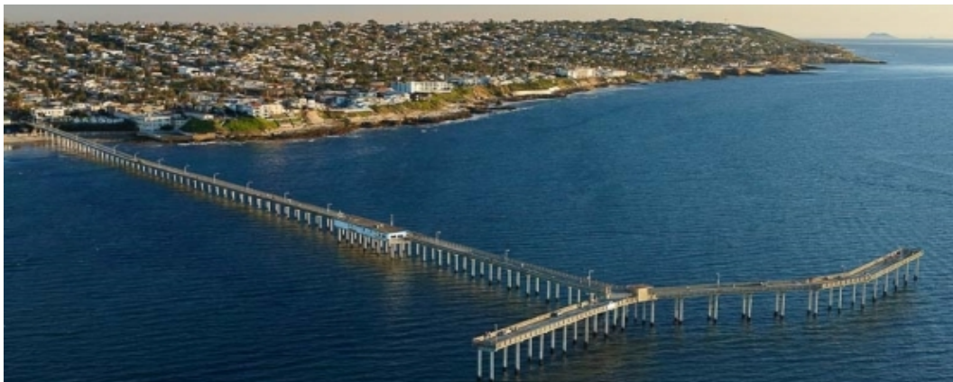
Current Ocean Beach Pier has exceeded its useful life.
