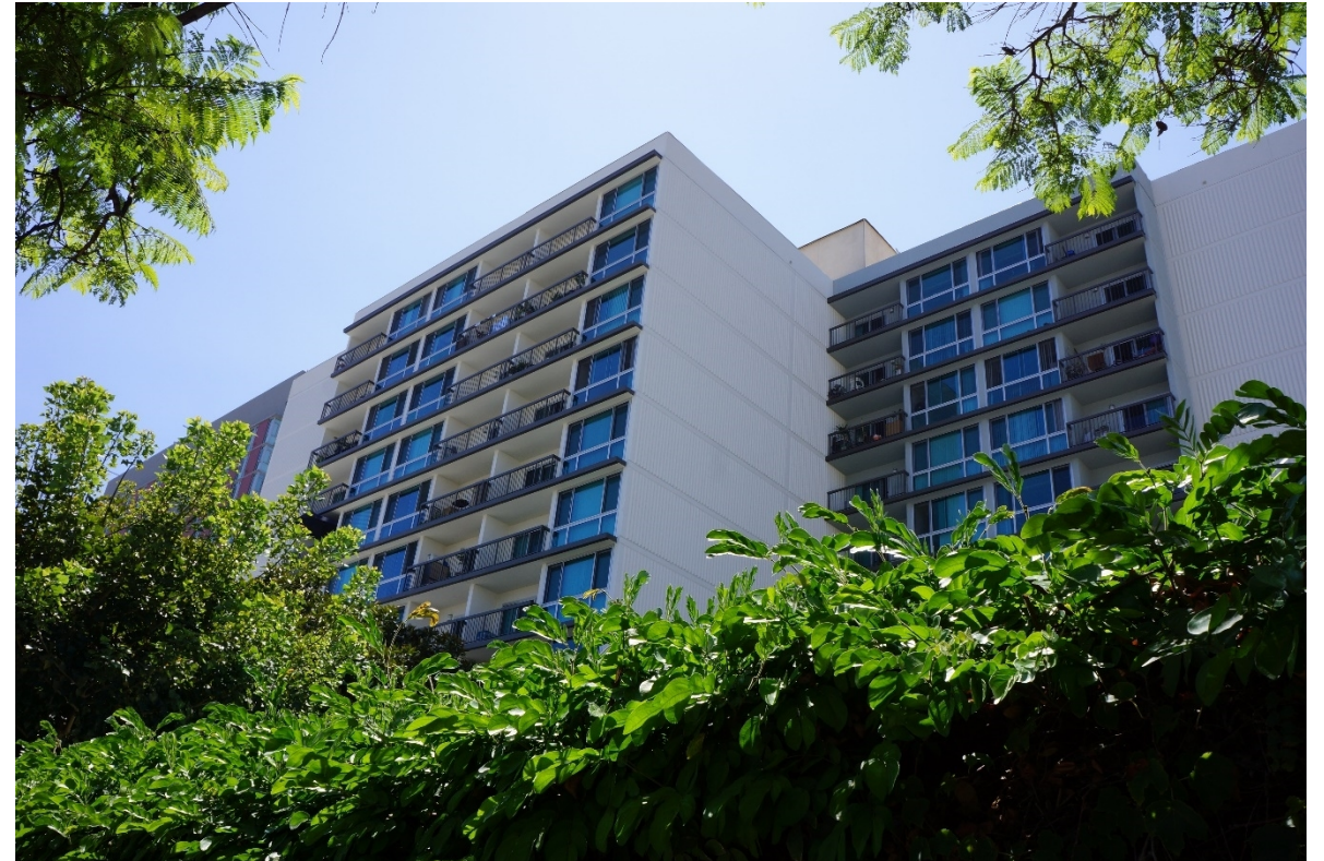
HDP collaborated with SDHC to acquire, rehabilitate and preserve the affordability of San Diego Square.
