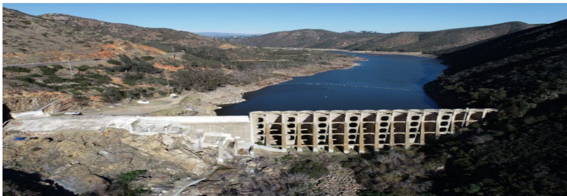
Existing Lake Hodges Dam
